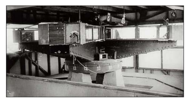
Figure 4. **Dayton Miller's light-beam interferometer,** at 4.3 meters across, was the largest and most sensitive of this type of apparatus ever constructed, with a mirror-reflected round-trip light-beam path of 64 meters. It was used in a definitive set of ether-drift experiments on Mt. Wilson, 1925-1926. Protective insulation is removed in this photograph, and windows were present all around the shelter at the level of the interferometer light-path. [8]
